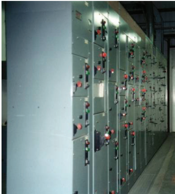
Figure 1. Motor control center (EPRI)
